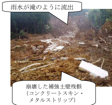
(c) 補強土壁残骸
